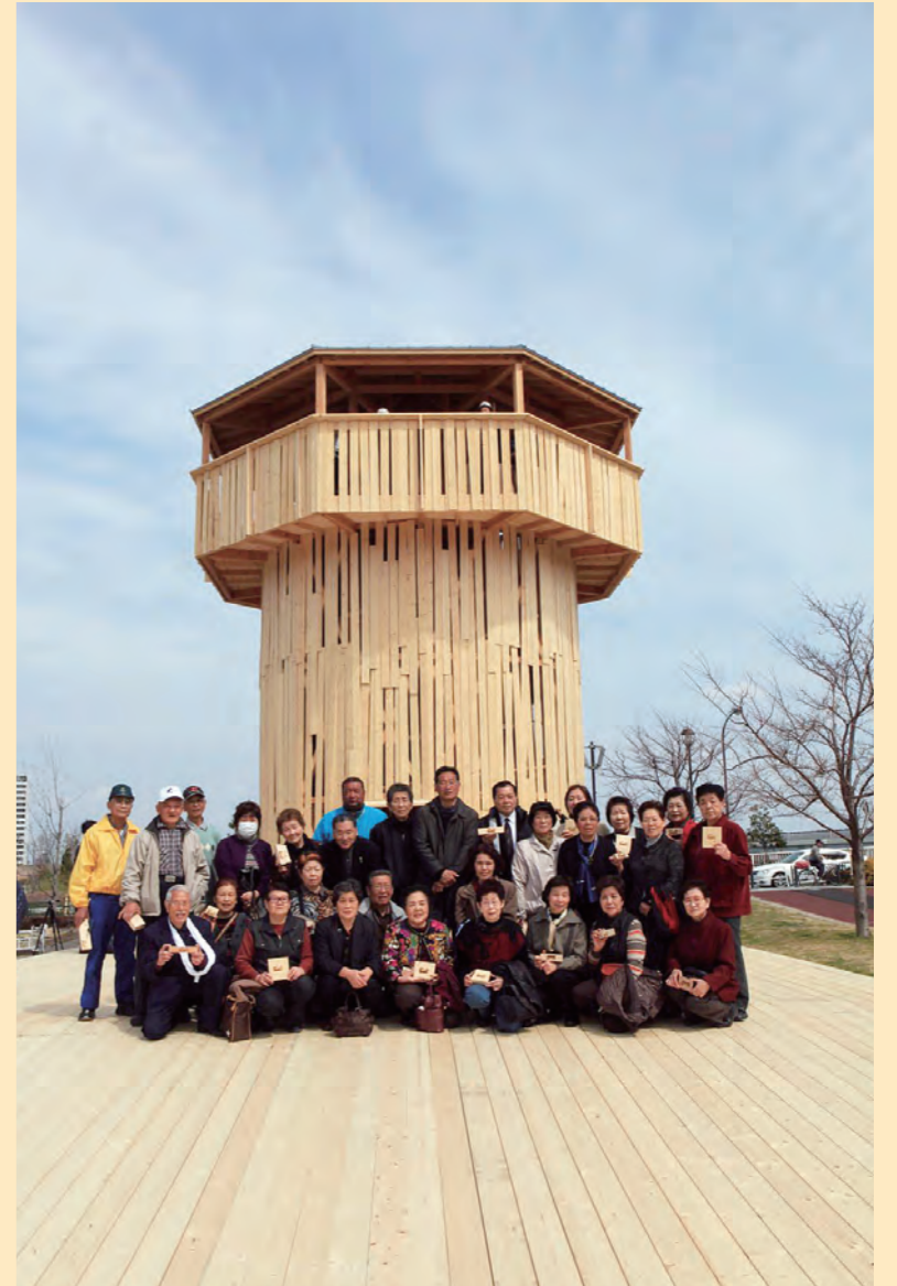
3.20 竣工 Construction Completed
